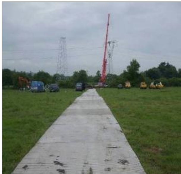
Figure 21 - Temporary Aluminium Panel Tracks
