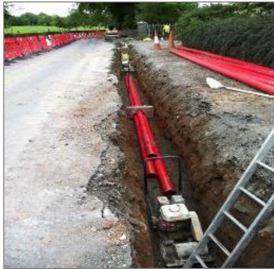
Figure 2 - 110kV Underground Duct Installation
