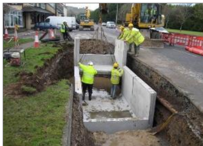
Figure 11 - Typical joint bay under construction (pre-cast)
