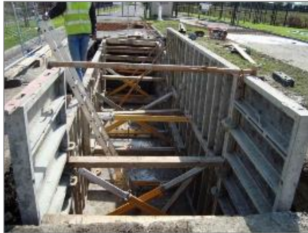
Figure 9 - Typical joint bay under construction (in-situ)
