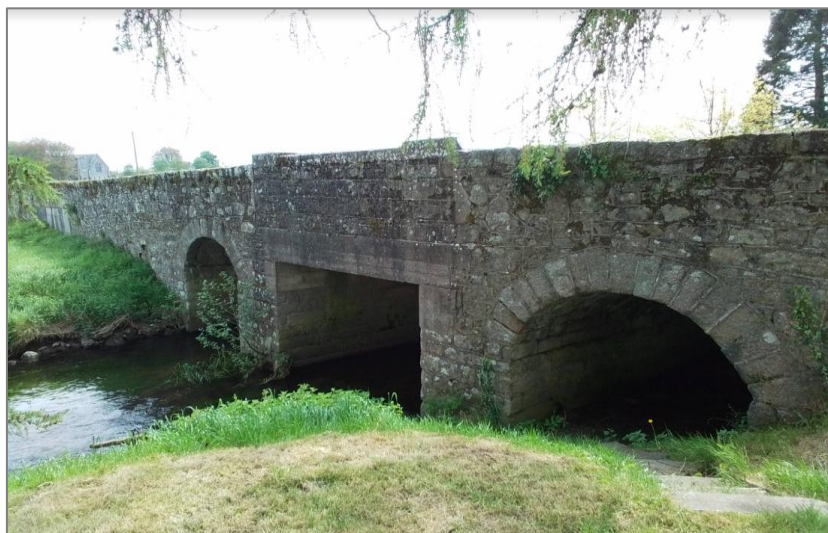
Figure 16 - Bridge 1 Rathoe Bridge
