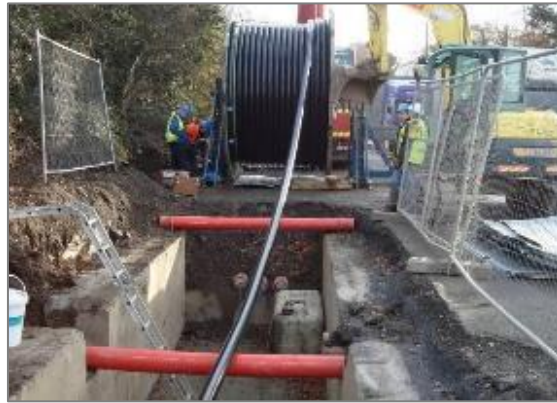
Figure 12 - HV cable pulling procedure (Typical drum set-up)
